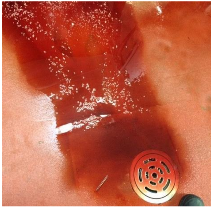
Typical inferior seal
