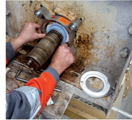
Second RotorCup and End cover installed
