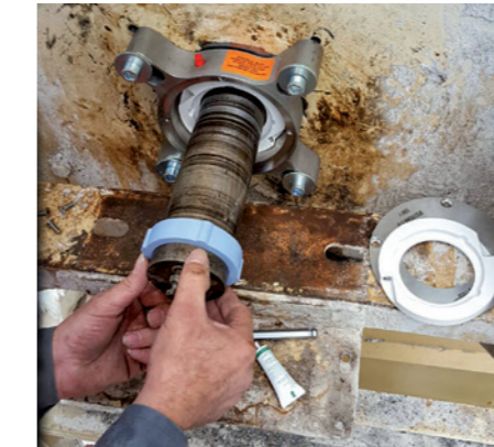
RotorCup and RubberBoot installed
